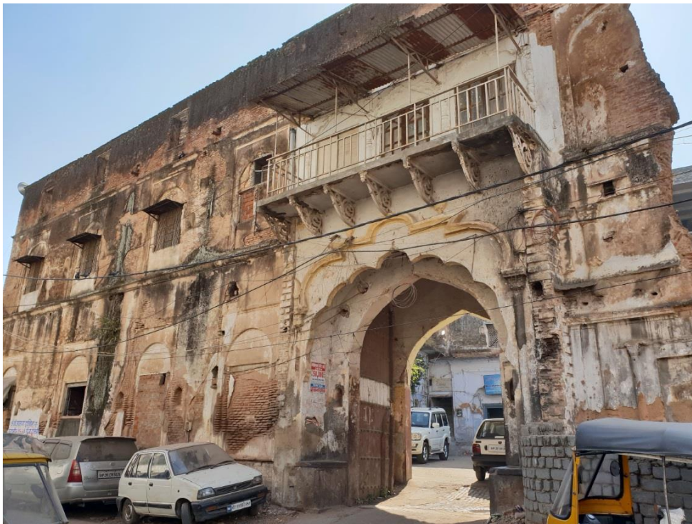
Figure 1. Bhopal, Peer Gate area. Mirroring destruction elsewhere, urban heritage is currently under serious threat in cities throughout India. Here, a Moghul influenced former courtyard house has lost its original inner complex and the right hand portion has been demolished pending redevelopment. (Source: Carsten Hermann)
